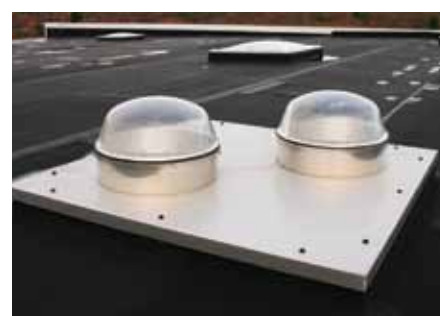
Bespoke flashing for skylight replacement (not a Solatube product)
